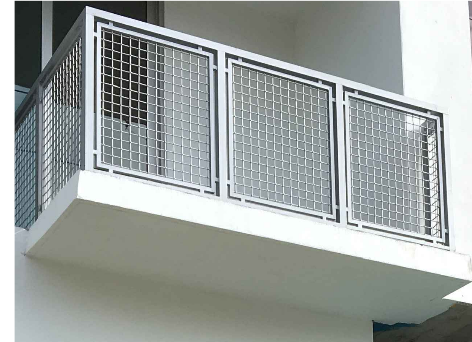
3 PERFORATED METAL MESH RAILING
